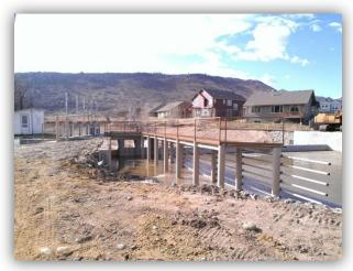
Figure 3 – Repaired ditch company diversion and headworks
